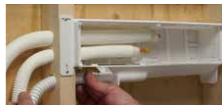
6. Insert pipes and drain hose
