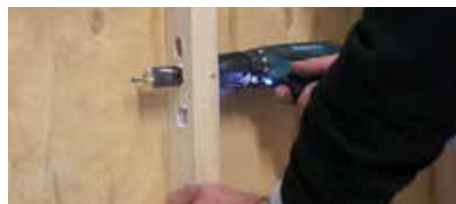
1. Drill holes in the structure for pipes
