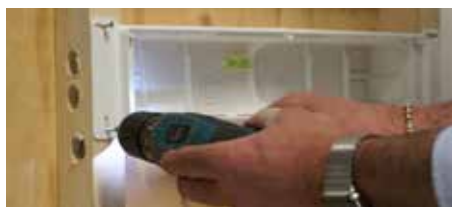
5. Fix box to the structure using screws
