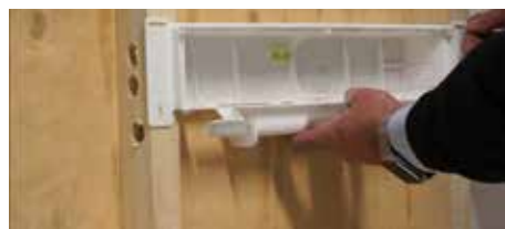
4. Place and align the box to the holes
