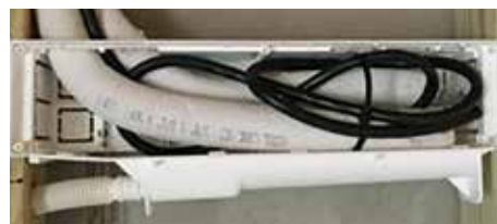
7. Insert wiring and connect drain
