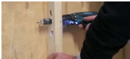
1. Drill holes in the structure for pipes
