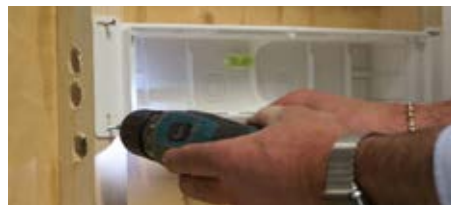
5. Fix box to the structure using screws
