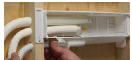
6. Insert pipes and drain hose
