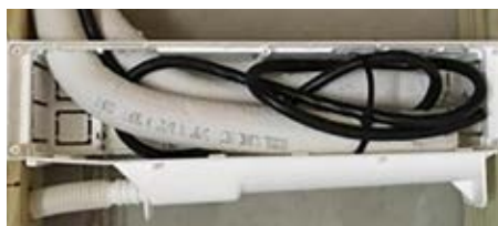
7. Insert wiring and connect drain
